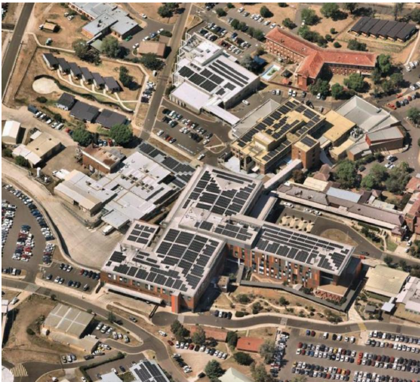
Figure 2: Aerial view of Tamworth Hospital
